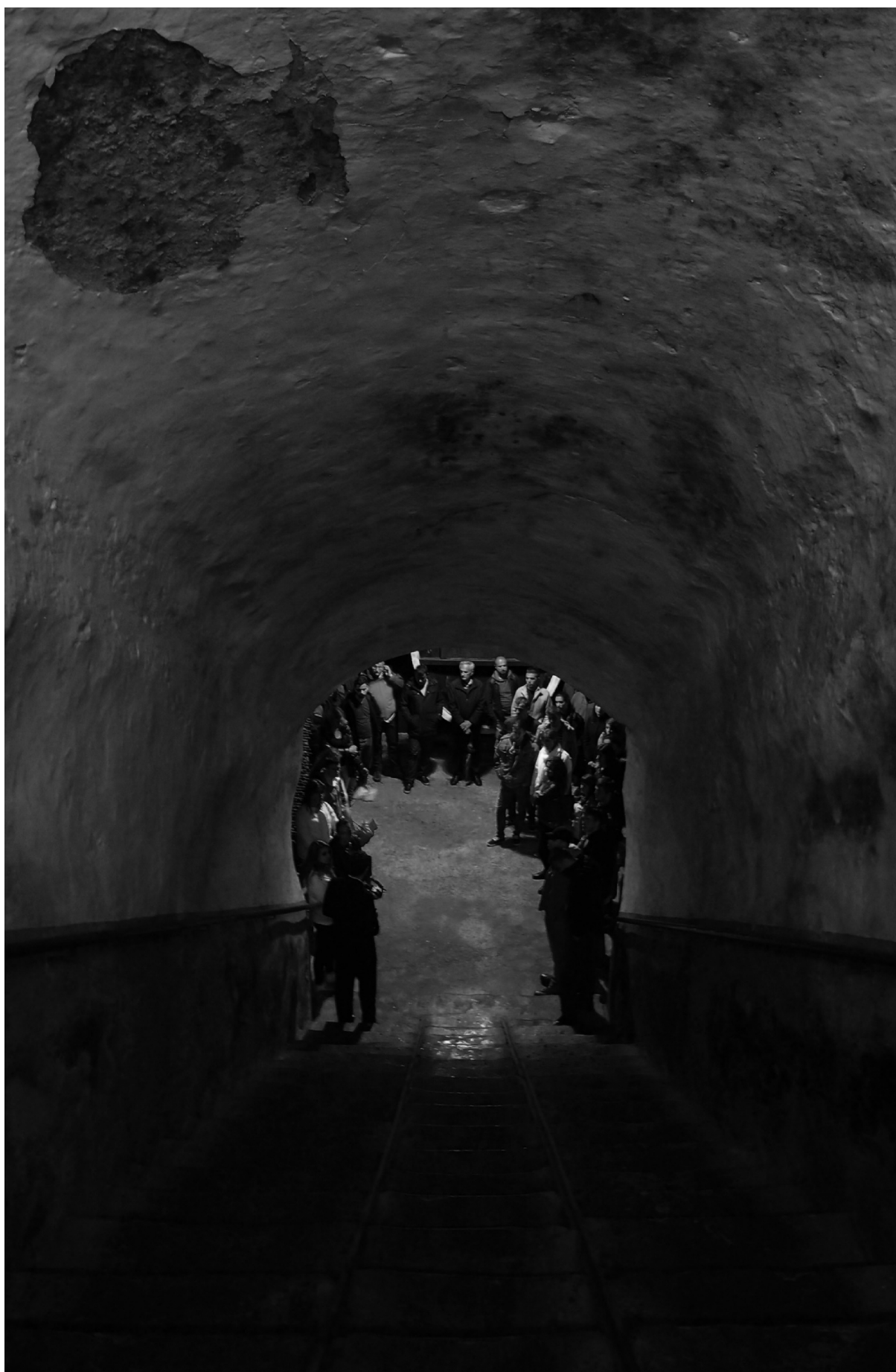
Photo 039. The entrance to the basement / Ulaz u podrum
